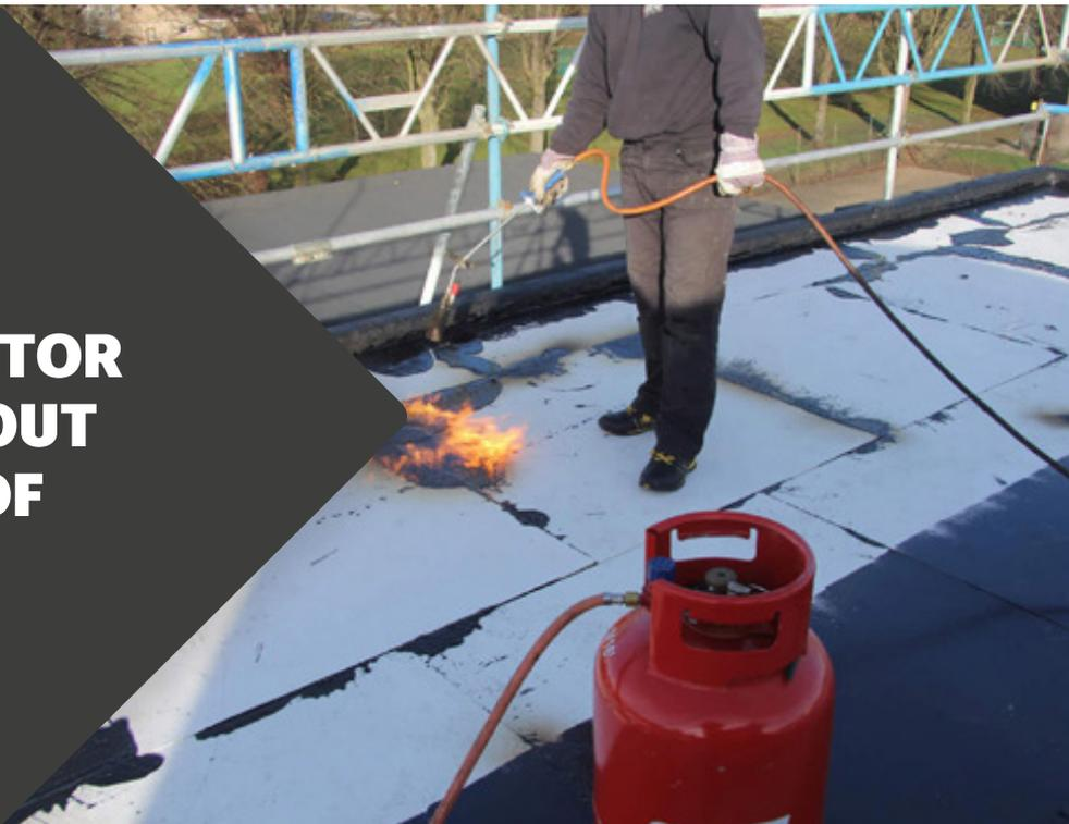
A Colchester based roofing contractor has been using Magply Recovery boards as part of a high specification build up, which provided its operatives with a relatively quiet as well as safe means of carrying out reroofing works to school classrooms during lesson times.
